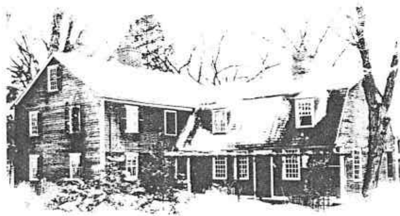
The Homestead. Home of Captain and Mrs. William C. Skinner. The present home is made of two combined houses, the front half being the original Newell home and the rear half being the original Woodford home. Both probably built in the 1660's.
